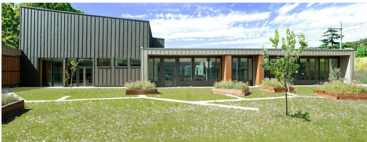
Figure 6 : Ecole Quai Pasteur – © Composite Architectes
